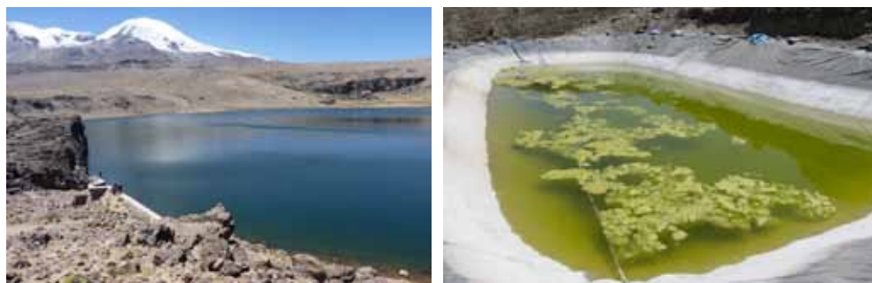
Figure 10. Open water storage behind a check dam (a) and in a plastic lined pond (b) in the Andes, Peru (Photo: Acacia Water).
