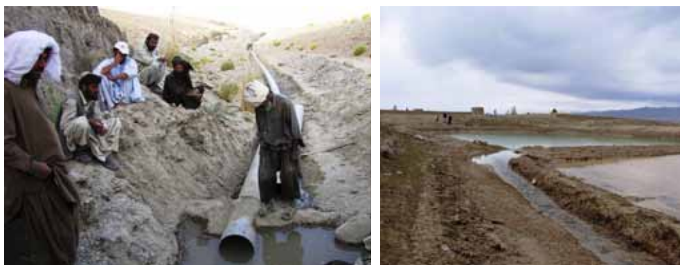
Figure 22. a) Villagers taking rest during improvement of the Qilla Iskan Khan karez system. They are installing a 30 cm wide PVC infiltration pipe inside the karez; b) The constructed geo-membrane reservoir (Photo: IUCN Pakistan, 2011 and 2010).
