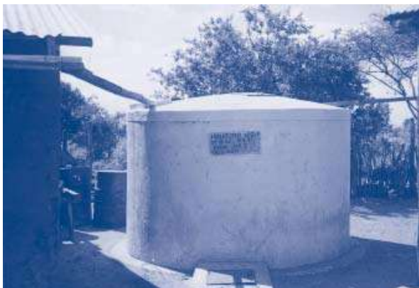
Figure 1.21 Simple roof catchment and storage. Source: IRC.
