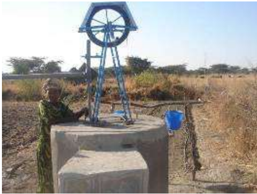
Figure 1.11 Well with rope pump
