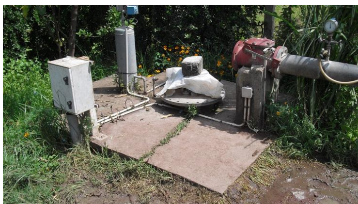
Fig. 9: Scope for improving wellhead protection
